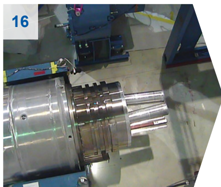
16 Pulling out the old plug.
