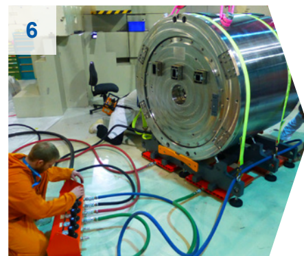
6 Moving the new beam plug on air cushion.
