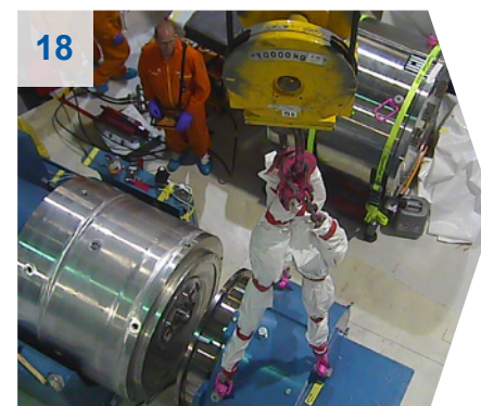
18 Dividing the old plug for the transport.
