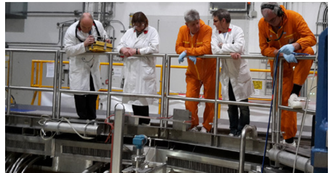
Fig. 3: J. Molch (FRM II), A. Debnar-Beinssen (Westinghouse), J. Werth, H. Hottmann (both FRM II), H. Bergh (Westinghouse), from left, have a keen eye on the installation in the reactor pool.
