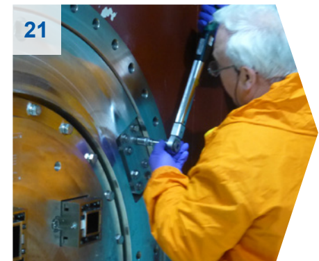
21 Fitting the new plug into the beam tube.
