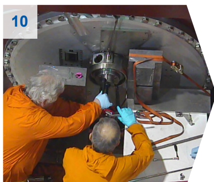
10 Dismounting the old plug's gear box.
