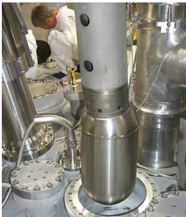
Figure 3: The moderator of the hot source in the reactor pool of the FRM II during installation.
