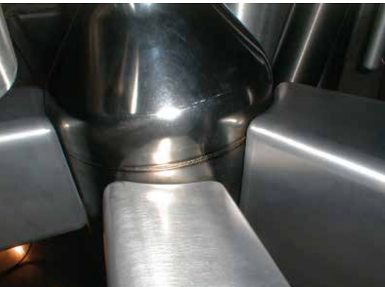
Figure 1: The cold source vessel surrounded by the beam tubes SR 1, 2, 4. View into the moderator tank of the FRM II before operation.
