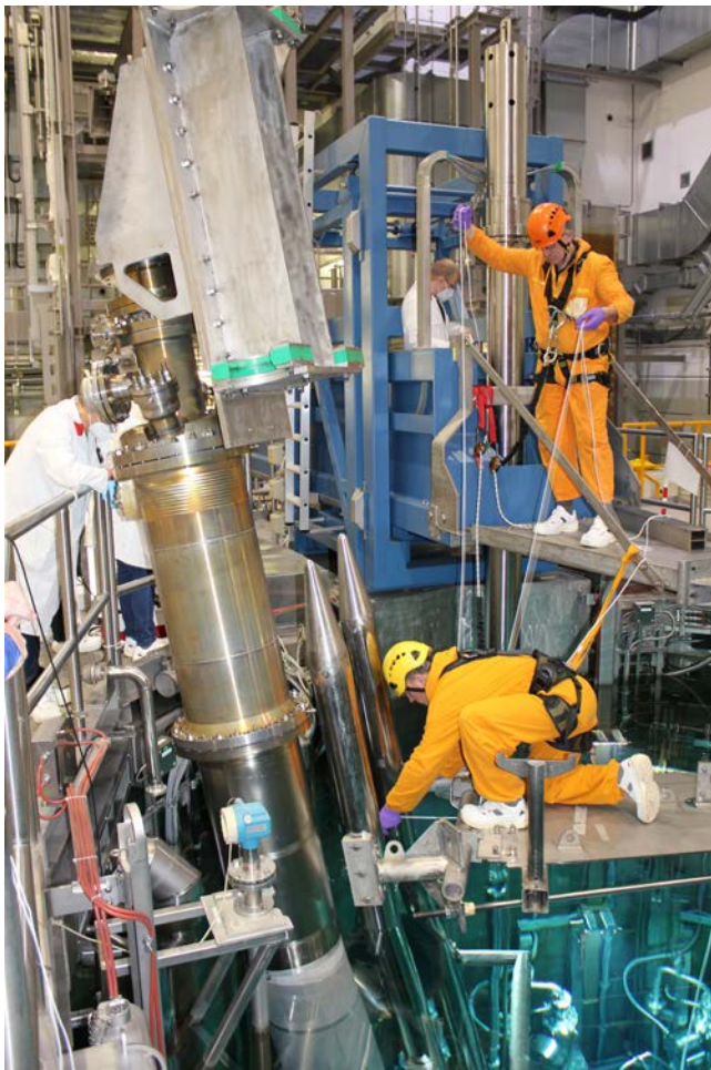
Fig. 1: The inpile section of the cold neutron source is being pulled from the moderator vessel (left) and placed for intermediate storage in the spent fuel pool (right).
