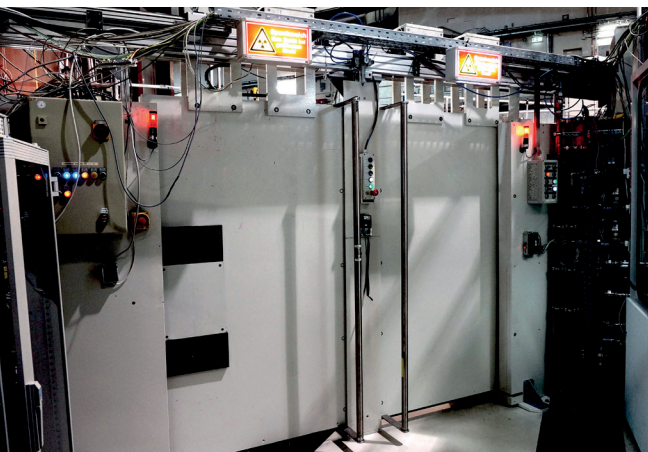
Fig. 1: The neighbours' doors: On the right access to the instrument POLI, on the left to HEiDi.
