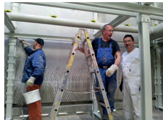
Fig. 2: Crew doing maintenance in the cooling tower (S. Zahn, M. Schulze, S. Hosszu, from left to right).
