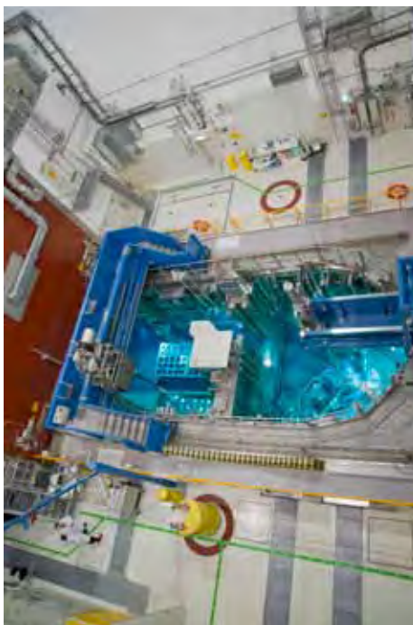
A look into the reactor pool.
