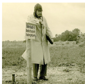
Figure 1: Prof. Dr. Tasso Springer in the year 1956 at the beginning of the construction of the FRM, the first German research reactor at Garching.
