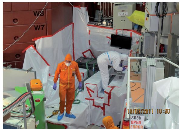
Fig. 4: Construction work at the HEiDi site during the reactor shutdown in March 2011.
