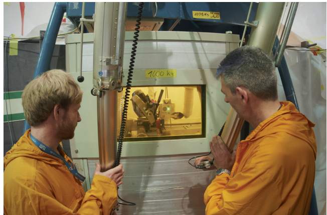
Fig. 3: Michael Schulz (l.) and a contractor working at the temporary hot cell in the experimental hall to dismantle parts of the beam tube SR11.
