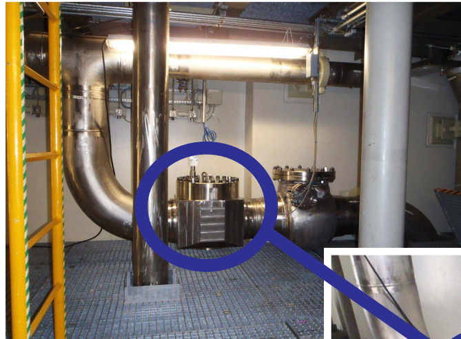
Fig. 1: The new second check valve.
